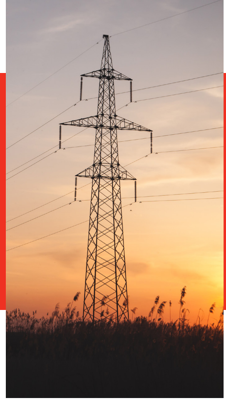
Figure 3. Example of a Tall Structure
